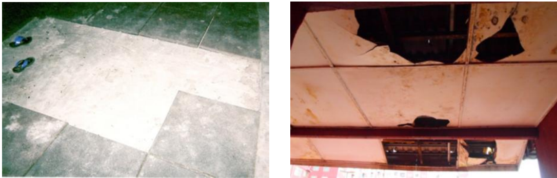
Fig. 7 & 8. Missing floor slabs and damaged ceiling (photos taken by author)
