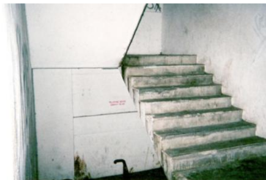
Fig. 9. Staircase with no railings (pictures taken by author)
